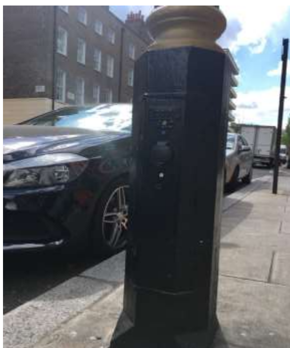
Examples of chargepoints retrofitted into existing lamp columns
