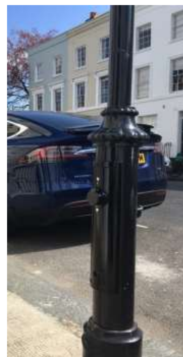
Examples of chargepoints retrofitted into existing lamp columns
